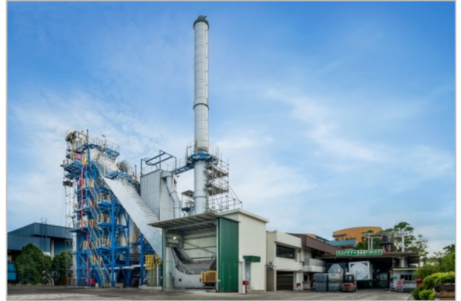
Appearance of TEC New Incinerator
